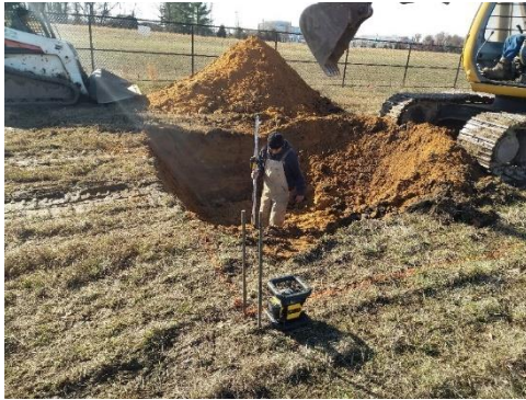
(c) Depth Check when Excavating
