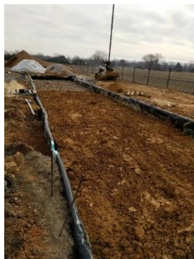
(a) Subgrade Layers Placed
